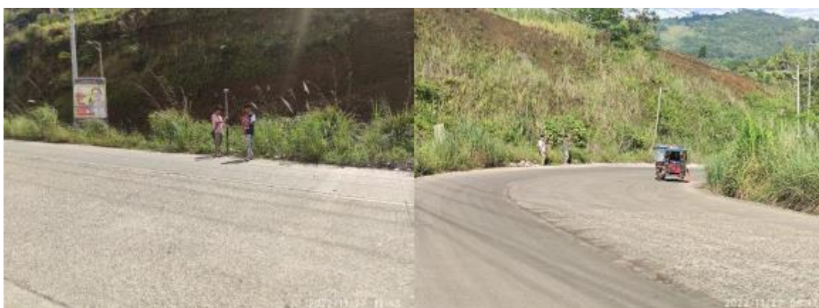
Figure 4. The image shows the shoulder covered with grass and other vegetation
